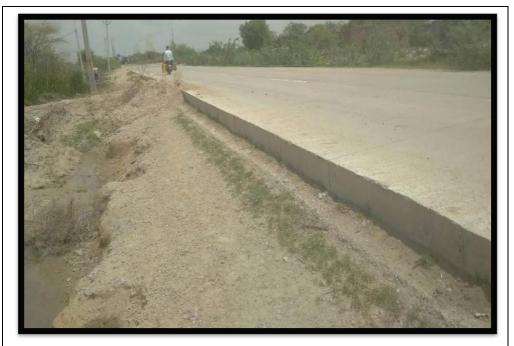
Image 1: Missing interlocking blocks/GSB shoulder/drain
